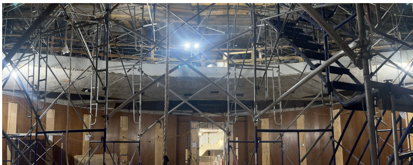
Main Sanctuary renovation underway.
